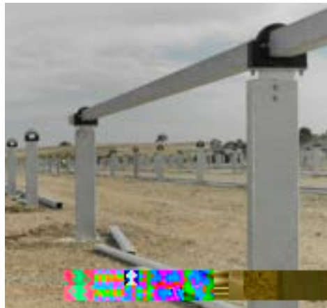
Spherical bearing installed in Zuera 11 MW, Zaragoza
