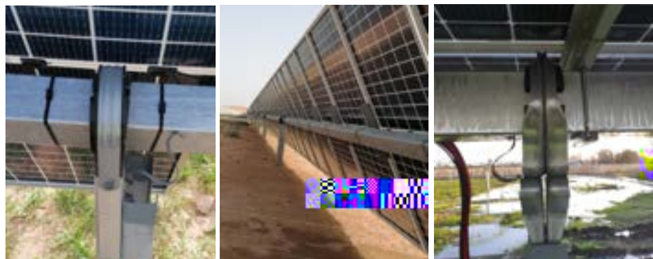
TrinaTracker roller bearing assembling example
