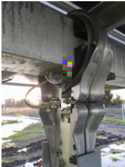
Lower bearing assembly in rd 2P
